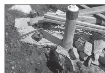
Figure 1. The slab around this capped well must be kept to keep water from entering the well bore hole.
