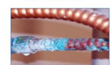
Figure 1. Corrosion at a connection on a water heater indicated by the blue-green color.
